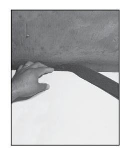
Acoustic Foam is simple to install for head of wall applications. Compress the Acoustic Foam into the joint between the top of the wall and bottom of the deck. The Acoustic Foam can be recessed into the joint or installed flush with the outside surface of the wall. Joints are butted together. No mechanical fastening of the Acoustic Foam is required.
