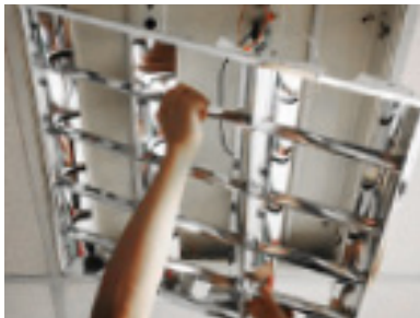
1. Remove the lens or louver (if required).
