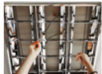
6. Replace lens or louver, if needed.
