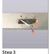
Attach the bracket to junction box using the 2 screws (provided). Pull the AC cable with connector through the bracket center hole.
