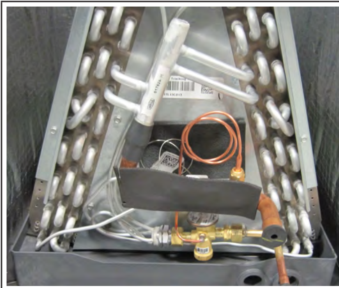
FIGURE 12. Insulated TXV Sensing Bulb
