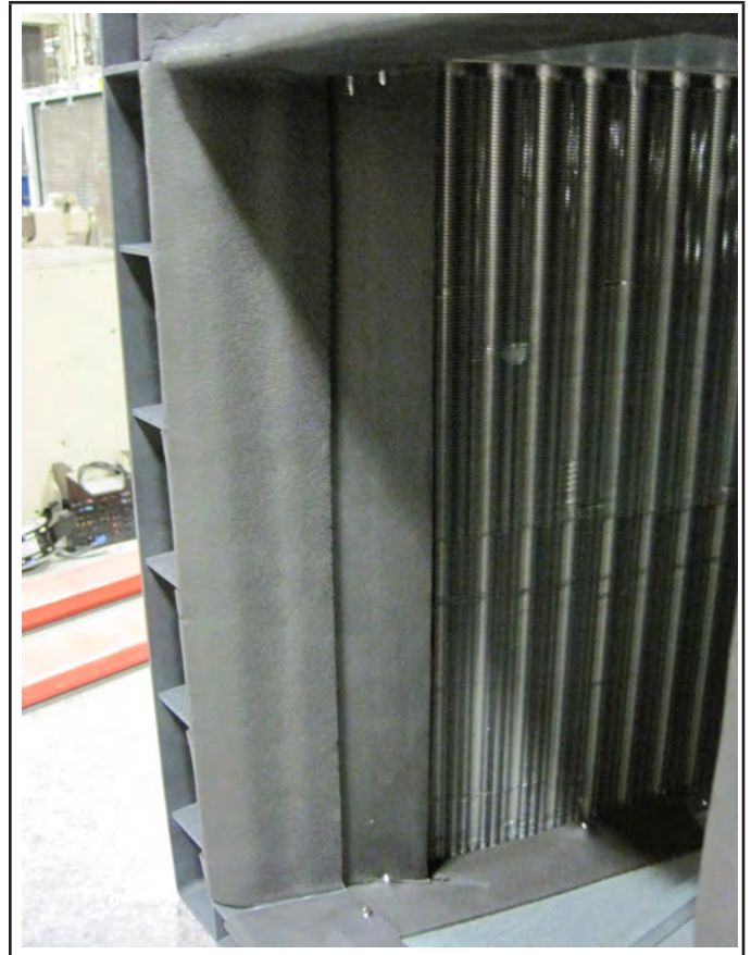
FIGURE 9. Insulated Drip Shield Installed
