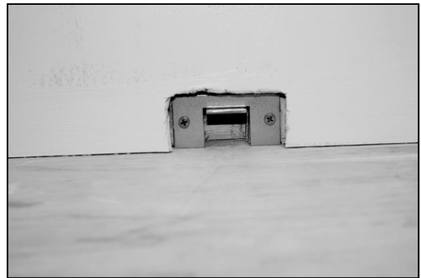
Install Nail Plate
