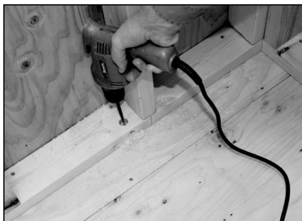
Drill Vertical Hole
