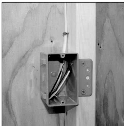
Mount Electrical Box
