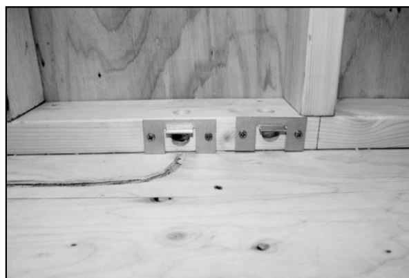
Install Nail Plate
