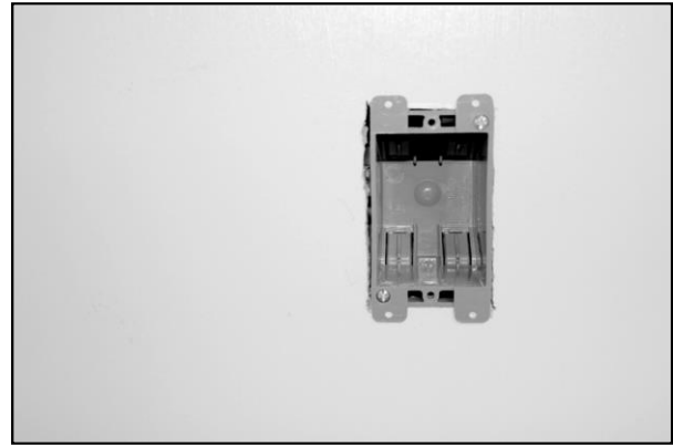
Install remodel J-box
