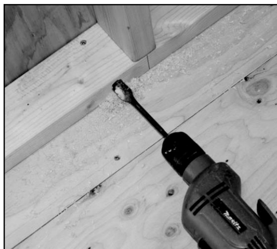
Drill Horizontal Hole
