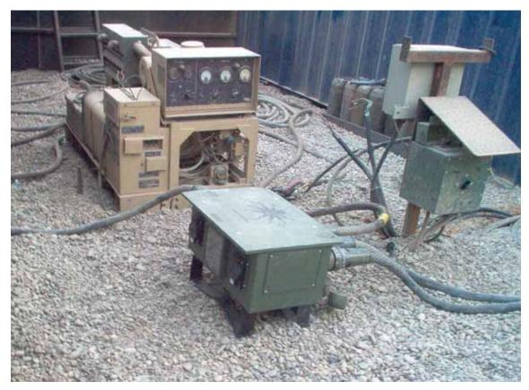
FOB/TOC Power Distribution (100 AMP) Using Mil Type 1068 Oscar™ Box
